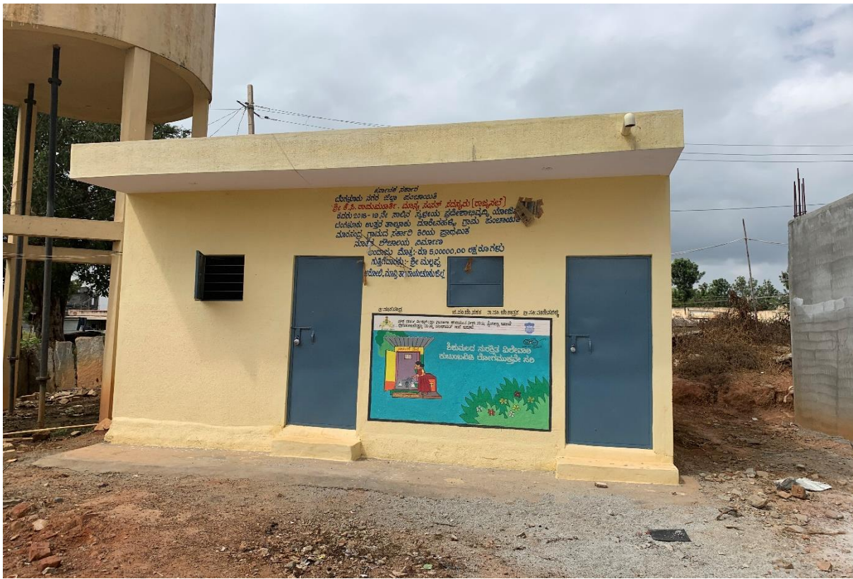
Toilet Constructed under Regional Development MP Funding estimated
